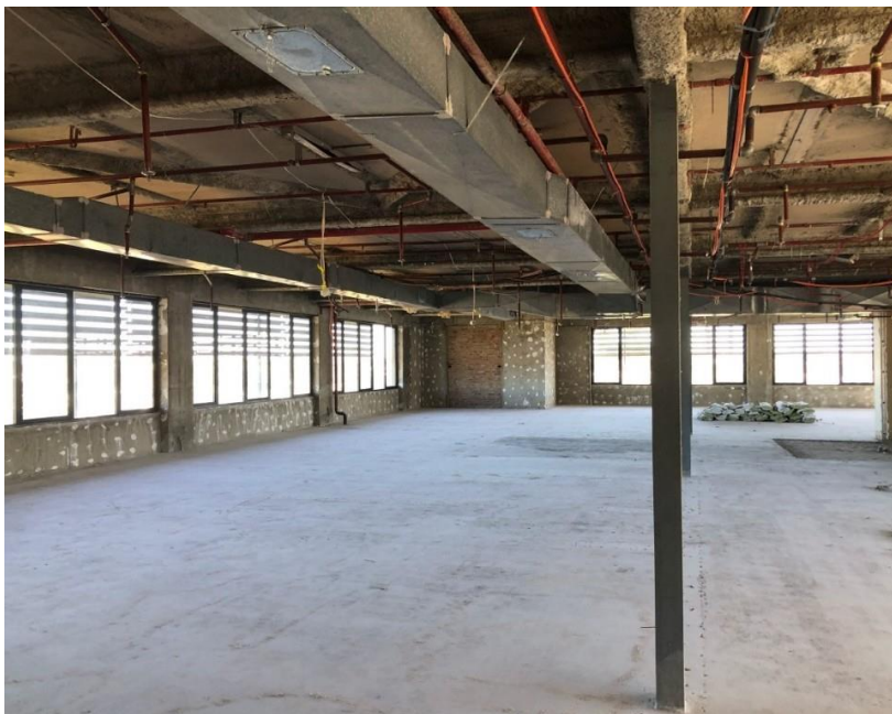
Figure 10: Internal view of strip out works
