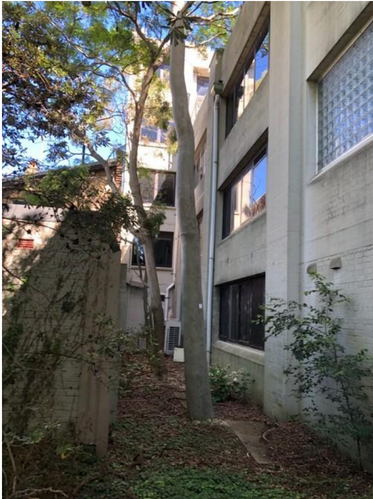
Figure 9: View along rear southern boundary
